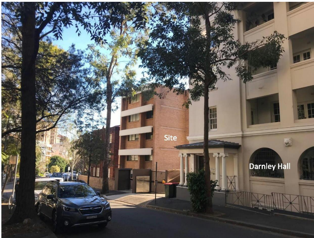
Figure 2: Site viewed from Onslow Avenue looking north
