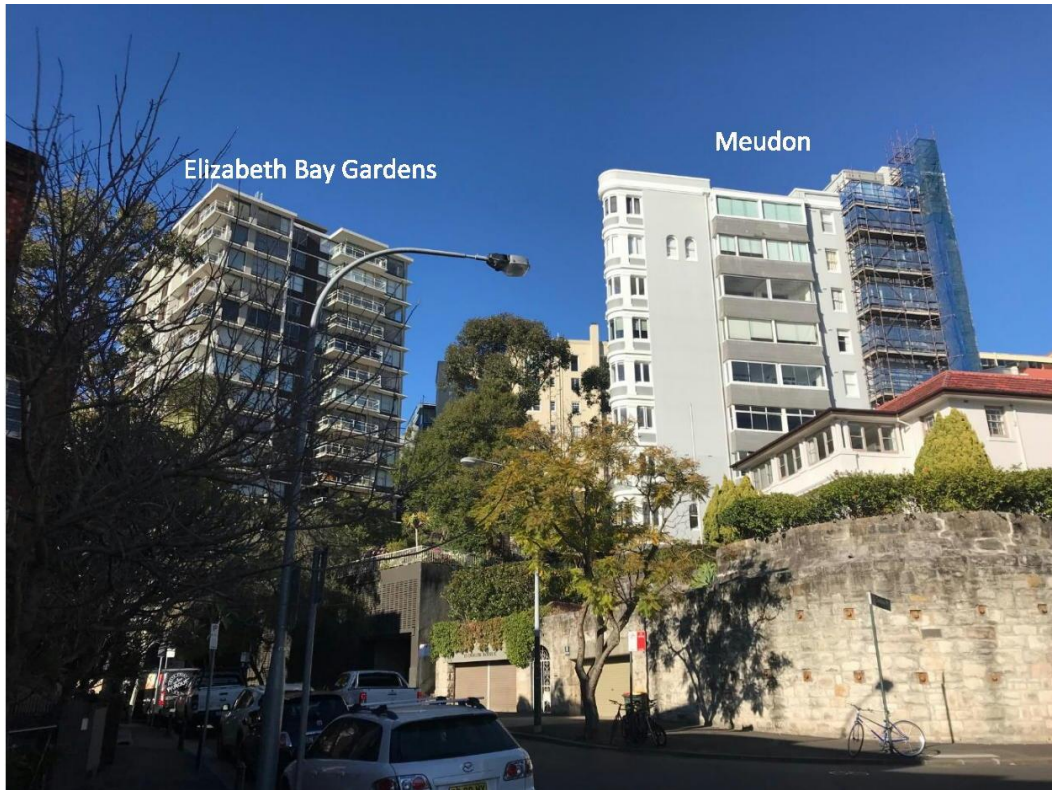
Figure 5: View looking south from top of Arthur McElhone Reserve towards the Meudon and Elizabeth Bay Gardens buildings
